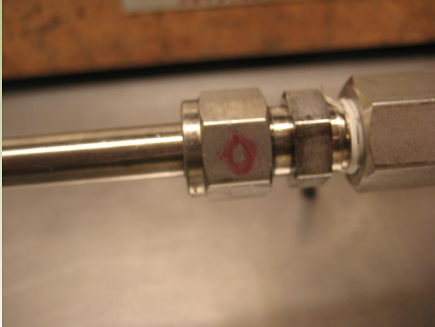
Assembled Test Connection (Typical) Prior to Pressure Test
